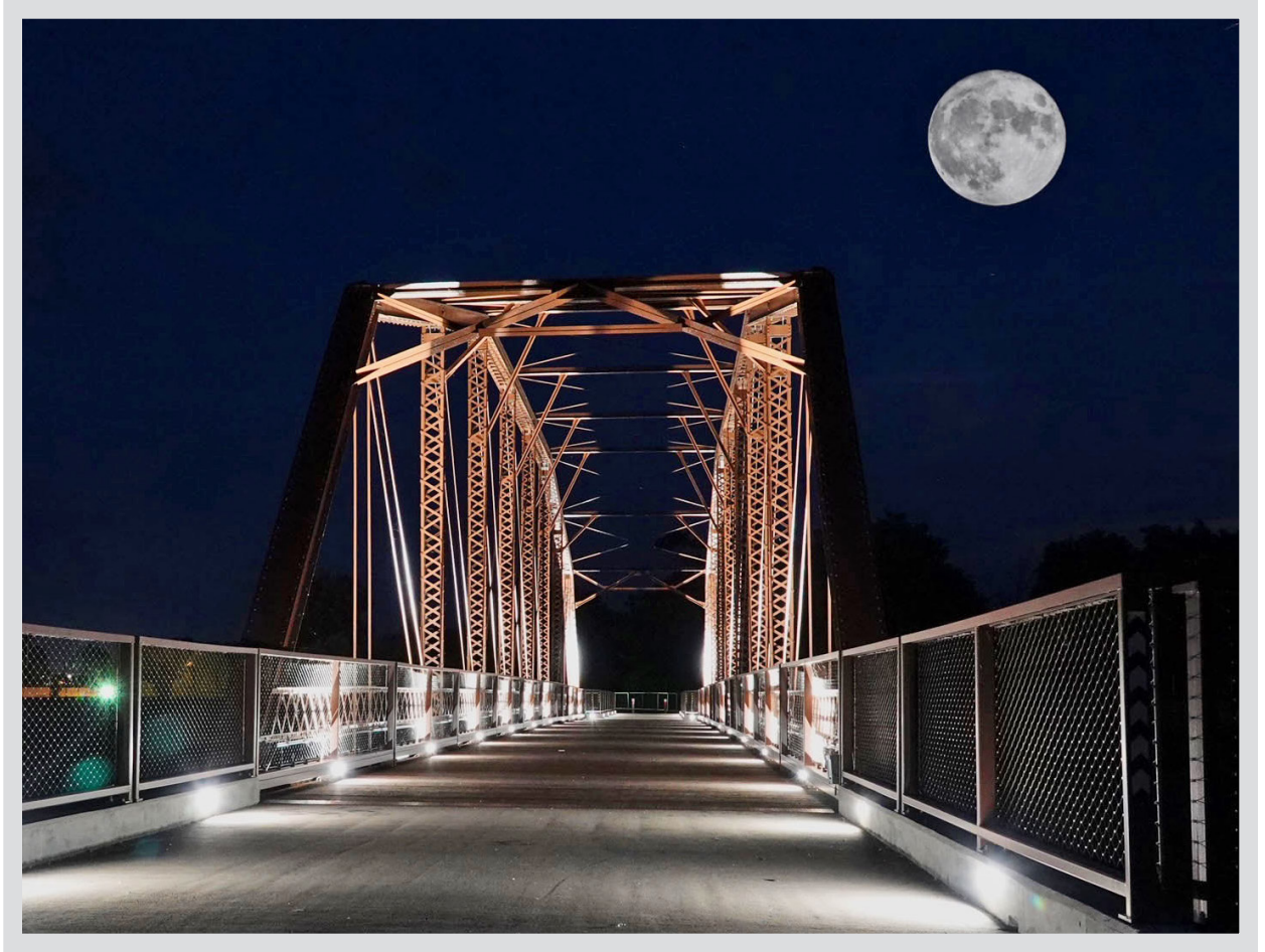
Kitselman Gateway Bridge Project
